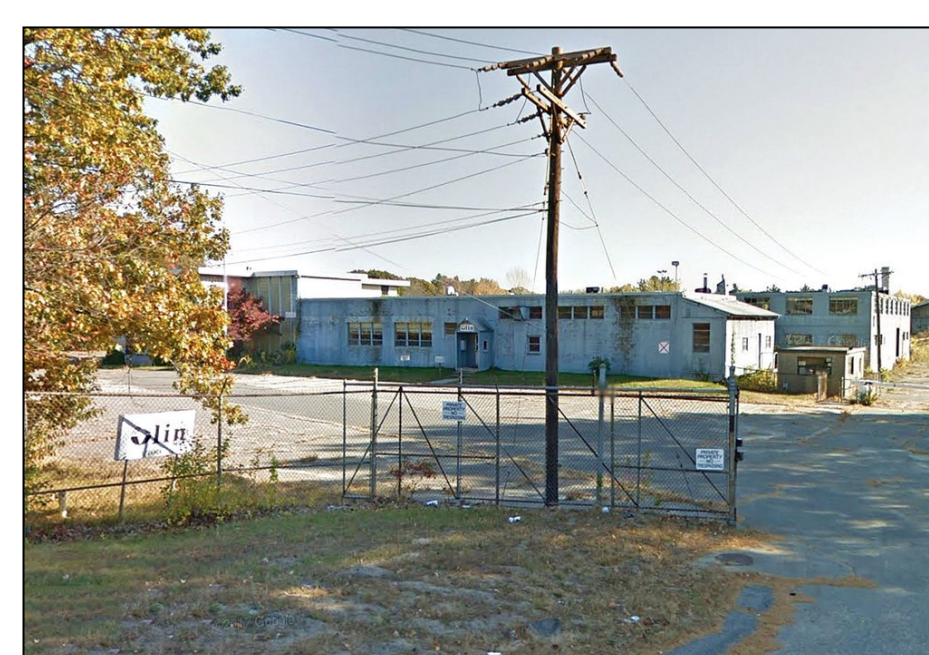
Olin Chemical Superfund Site Wilmington, MA
